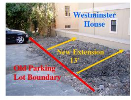
trench between the back parking lot and the retaining wall with Westminster House. To date, there have been 40 truckloads amounting to about 60 cubic yards of backfill. The acquisition of this sizeable area will add 5 more parking spots to the lot, which in turn increase revenue from parking on game days. Jake also plans to repaint the parking spots when the extension is finally completed.
